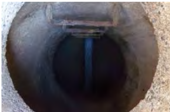
Manhole Before Install
