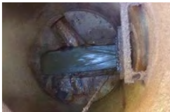
Manhole Before Install
