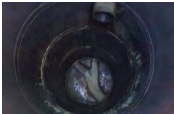
Manhole Before Install
