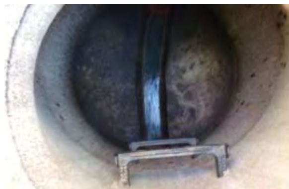
Manhole Before Install
