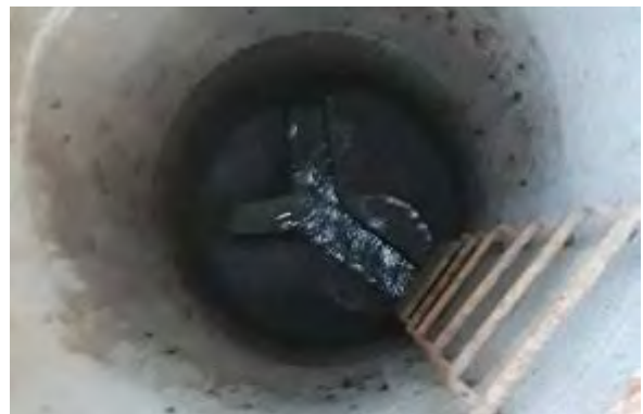
Manhole Before Install
