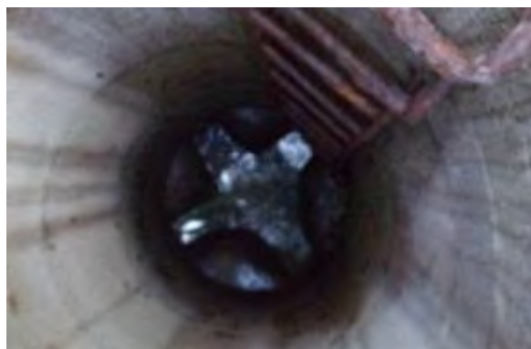
Manhole Before Install
